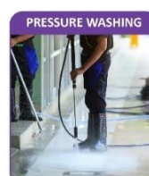
PRESSURE WASHING Apply by the foam generating equipment. Wash off using pressure washing.
